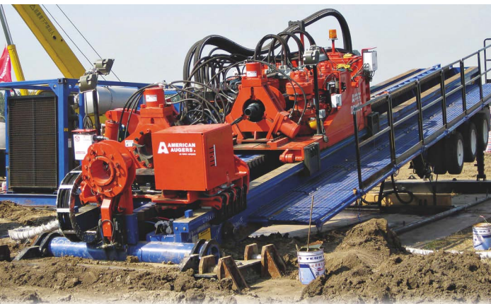
A brand of Astec, American Augers offers eight HDD models above 20,000 pounds in maximum thrust and pullback. The range is topped off by the DD-1100, which according to data compiled and verified by Spec-Check boasts the largest rated thrust and pullback in the industry, at 1.1 million pounds.
